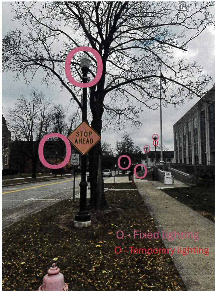
Figure 3: Picture of 6 fixed and 1 temporary light near the drop box.
